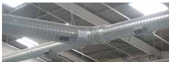
Suspended Air Ducts
