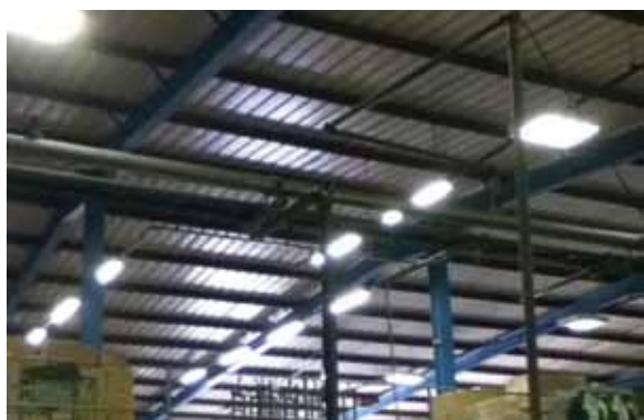
Lighting Unnecessary with Roof Lights
